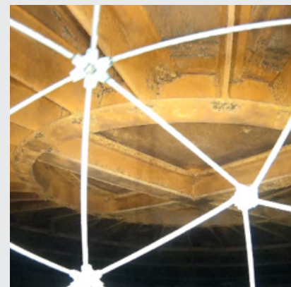
Roof visual inspection
