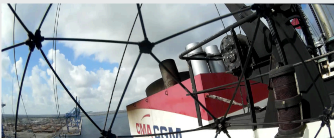
Exhaust Funnel Inspection
