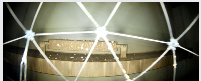
Anode integrity checking
